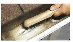
I Use a wire brush around the hole to clean and scuff the metal. Cut a patch from the same metal as the gutter.
