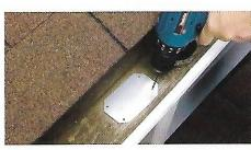
2 Set the patch piece in position, and drill pilot holes for pop rivets through the patch and the gutter.
