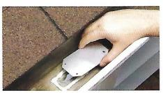
Caulk the area covered by the patch and the back of the patch with silicone, and press the patch into place.
