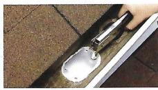
Secure the patch with pop rivets. Install as many as you need to make the caulk ooze out on all sides.
