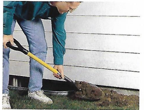
Turning a gully into a hill that slopes away from the building helps to take the strain off leak-prone foundations.
