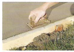
**II** Form the perimeter of the slab with an edging trowel. Run it slowly back and forth to smooth the mix and release the form.
