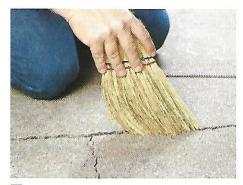
**II To make minor repairs** of small cracks, start by cleaning out dirt and debris with a whisk broom.
