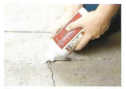
**2 Concrete repair caulk** provides a quick fix for minor cracks. It prevents further damage but is only a temporary repair.
