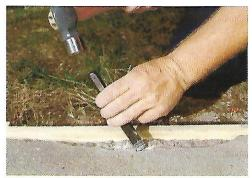
To patch larger areas and edges, clear out loose debris with a cold chisel. Add a form board to contain the patch material.
