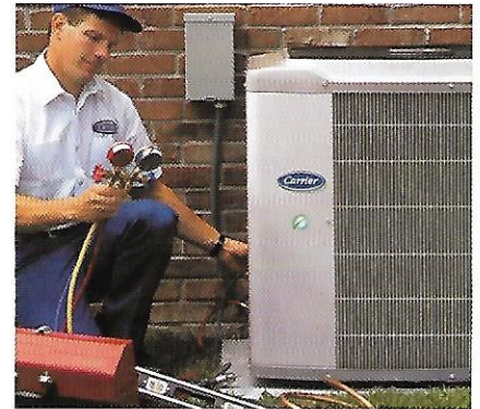
Homeowners can take care of basic maintenance, but you need a contractor to recharge the refrigerant.
